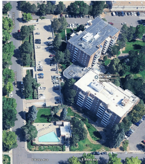
Figure 1: Aerial View of the Plaza de Monaco Parking Garage
