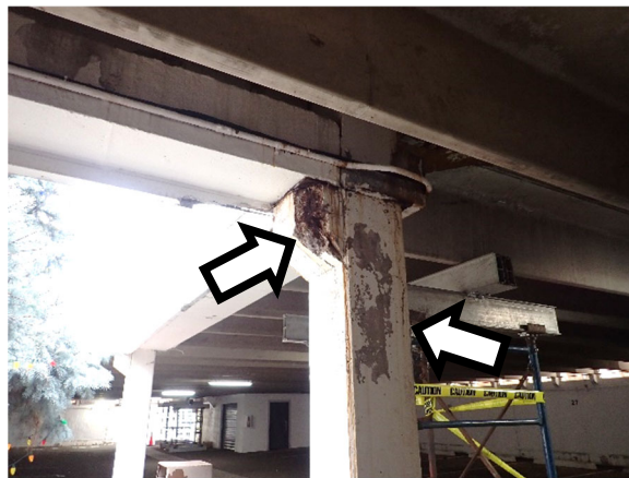
Photo 1 – Deteriorated Column
