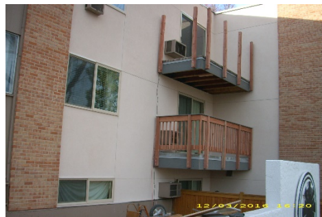
New Windows, railing, and stucco
